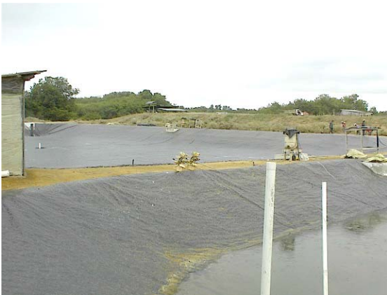
Two ponds lined with plastic.
